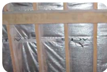
4. A totally airtight membrane
