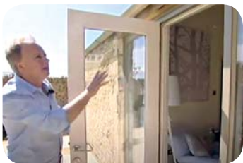
5. A tape seal around all the joinery
