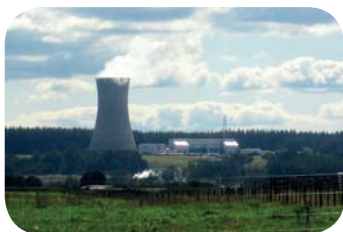
The Ohaaki Geothermal Power Station, New Zealand
